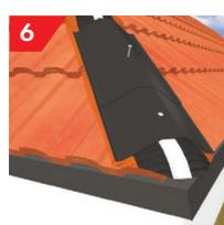
Cut the first hip support tray in half and to suit the eaves and secure in place using corrosion resistant nails. Overlap the next full support tray by 50mm, secure and continue in the same way along the length of the hip. The remaining half of the first tray can be used at the top of the hip. Please note, hip support trays are not essential for plain tile or slate roofs.
