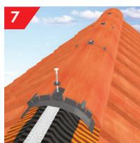
7 Place end ridge tile centrally over the white spine of the Roll Fix and insert ridge seal under and between ridge tiles. Secure using the 100mm screw, washer and clamping plate provided. Continue this process along the ridgeline to the abutment, hip or gable. All abutments and gable end ridge tiles require a second-point of mechanical fixing, usually achieved by drilling and securing to the ridge batten.
