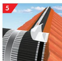
5 Starting at one end, unroll the Roll Fix centrally over the ridge batten, making sure there is 75mm cover on each side of the top course of tiles and sufficient to fold down at each gable over the batten ends or dry verge. Secure in place using corrosion resistant nails or staples at 300mm centres through the white spine of the Roll Fix. When joining Roll Fix, laps should be a minimum of 75mm.
