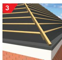
Screw fix 50 x 50mm hip battens to supports. The hip batten can be built up using 50 x 25mm tiling battens.
