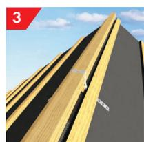
3 Fix top tiling batten as normal, ensuring a 10mm air gap remains.
