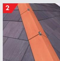
At the eaves junction at the base of the hip, a clay block end hip tile is recommended, which must be mechanically fixed into the hip batten to ensure a second mechanical fix.
