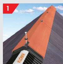
1 In principle the procedure for laying and fixing Roll Fix with Clay Plain Angle and Half Round Ridge Tiles on a roof is the same as for the fixing of concrete tiles. An exception to this rule is that a single 25mm hip batten may be sufficient for some angled Clay Plain Ridge Tiles. When using the KR5100 kit with 300mm clay ridge, the clay conversion kit (KR5100-6) is required.
