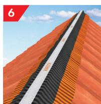
6 Remove release paper from the adhesive strip, dress neatly onto dry, clean and dust free tile surfaces, ensuring continuous contact with the tile but without flattening the aluminium rolls. Continue this process along the ridgeline. A continuous bead of Klobber Flashing Glue (product code PACCGGL) applied along the butyl strip can be used to install the ridge roll on a damp surface.
