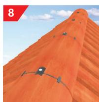
8 Once completed, the finished roof provides a mortar free ventilated ridgeline. Gable ends can be finished with a Klobber Ridge End Cap or a block end ridge tile.
