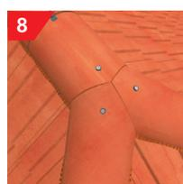
Once at the apex, close mitre both the hip and ridge tiles; drill and secure to the hip and ridge batten using the screws provided to ensure each cut tile has a second mechanical fix. To support the three mitred tiles, a small bed of mortar can be applied on top of the Roll Fix. The mitre junctions then require sealing with an appropriate roofing grade waterproof sealant. If Roll Fix is not used on the ridge, a lead or Wakaflex Lead Alternative saddle must be used under the mitre.
