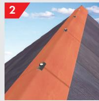
2 At the ends of the ridgeline, a clay block end ridge tile is recommended, which must be mechanically fixed into the ridge batten. A fixing hole will need to be drilled into the end of the ridge tile to allow it to be fully secured into the ridge batten and to serve as a secondary mechanical fix.
