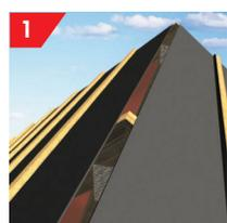
1 Install the underlay and battens as normal but leave the underlay 30mm short of the apex on both sides to allow ventilation. At this stage do not fix the top tiling battens. If no ventilation is required then the underlay can be carried over the apex if preferred.
