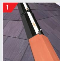
In principle the procedure for laying and fixing Roll Fix with Clay Plain Hip Tiles on a slate roof is the same as for the fixing of concrete tiles. An exception to this rule is that a single 25mm ridge batten may be sufficient for some angled Clay Plain Hip Tiles. When using the KR5100 kit with 300mm clay ridge, the clay conversion kit (KR5100-6) is required. When using the KR5001-1 with 300mm clay ridge, the clay conversion kit (KR5001-6) is required.
